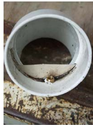
Photo 3 - Dilts water dam
